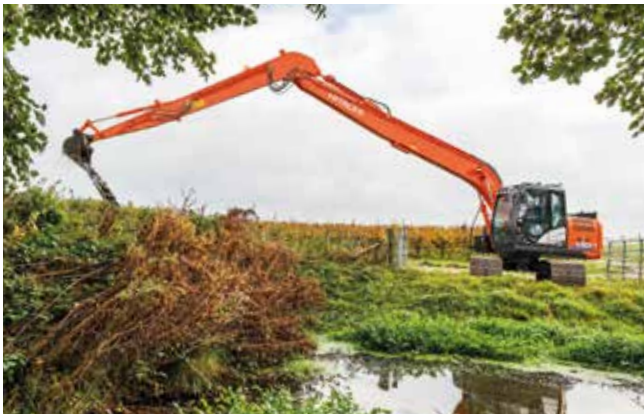
Special application excavators
